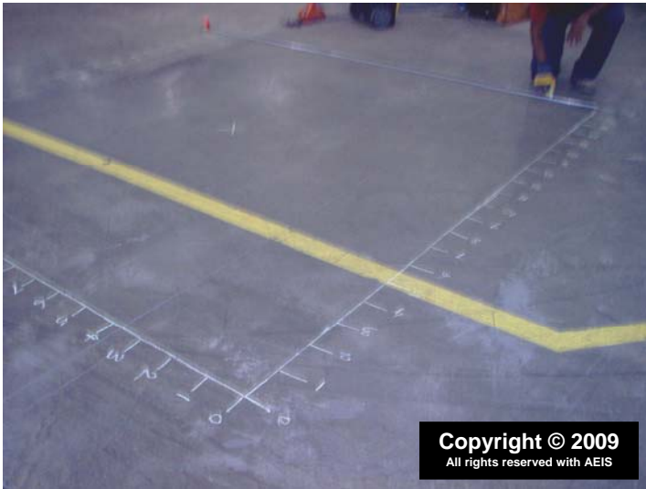
Figure 1: Grid lines were laid out in order to collect the data at closely spaced intervals in both directions.
