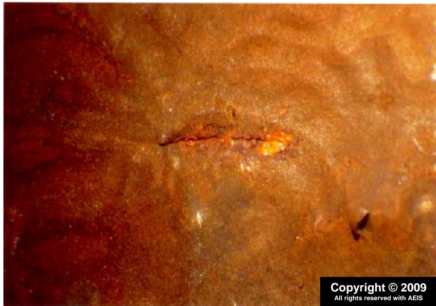
Figure 4: Another Crack Lip on the Inside Surface.
