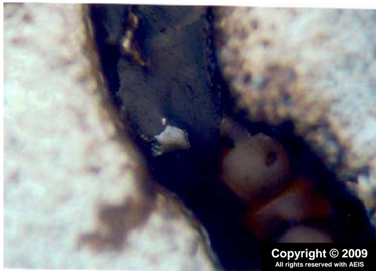
Figure 10: Slag on Internal Surface of the Crack near the Inside Surface
